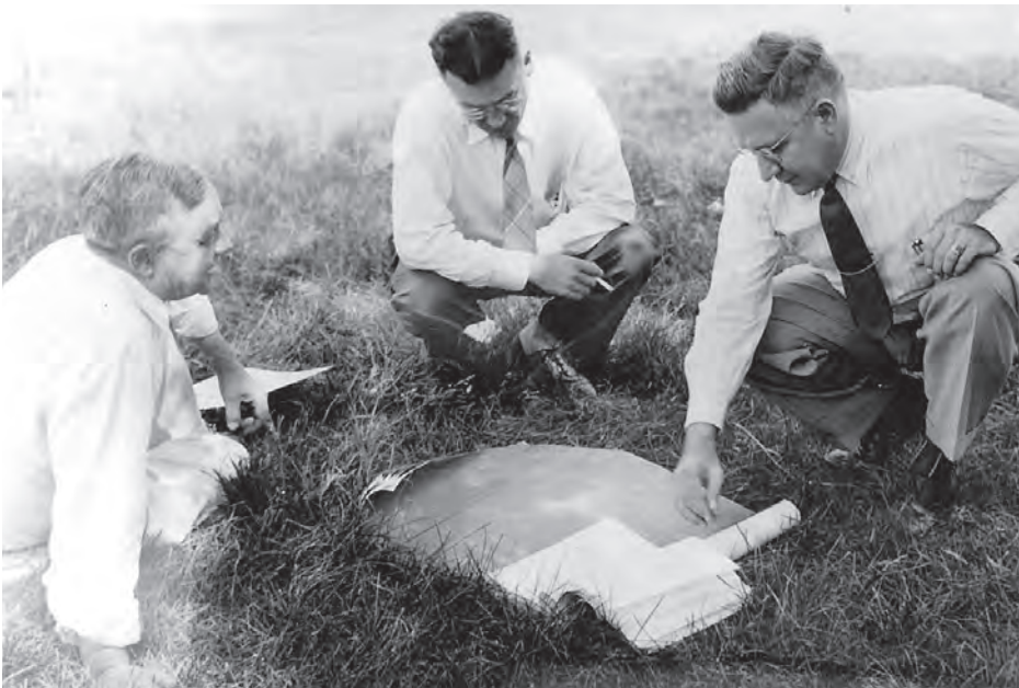
Architects and engineers from Weiler and Strang (including Joe Weiler on the right) meet at the site of the future Queen of Peace school in 1947 to discuss the design and construction of the new school.
